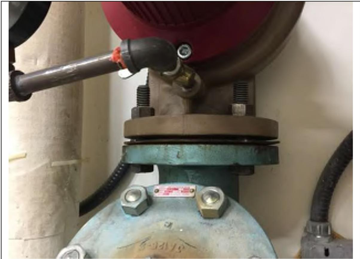
Picture No. 31: *Potential for asbestos pipe flange gaskets*
