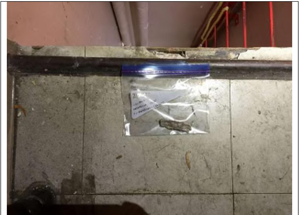
Picture No. 10: Non asbestos leveling compound beneath floor tiles (O1)
