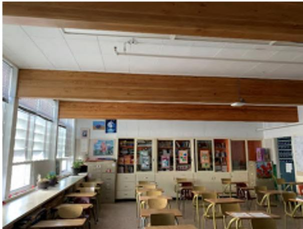
Photo #2 – Typical Glulam Roof Beams
