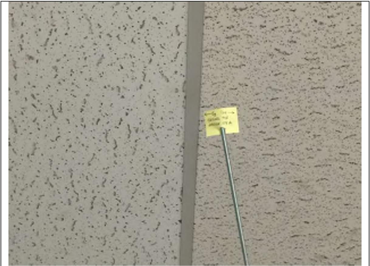
Picture No. 19: Non asbestos ceiling tiles (G3/G4)
