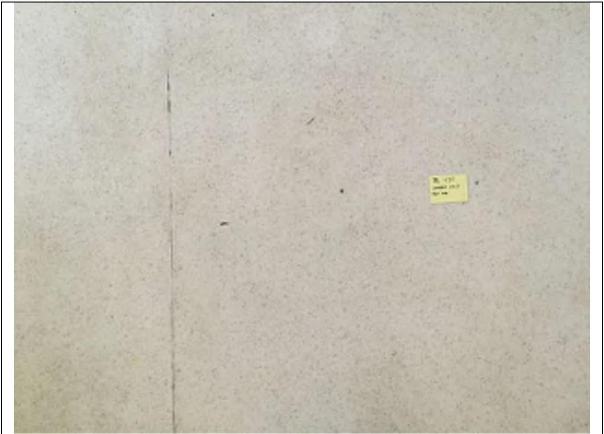
Picture No. 17: Non asbestos vinyl floor sheeting (I2)
