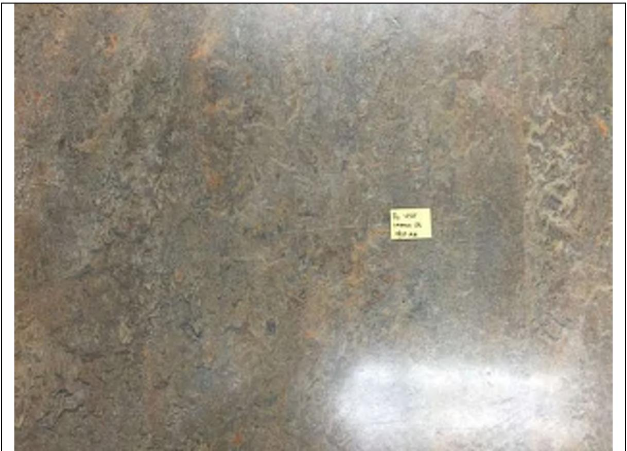
Picture No. 18: Non asbestos vinyl floor sheeting (I3)
