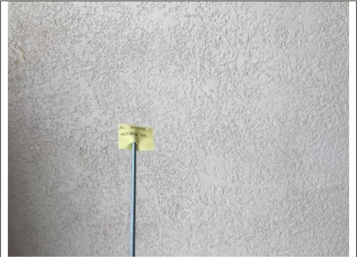
Picture No. 2: Non asbestos ceiling texture
