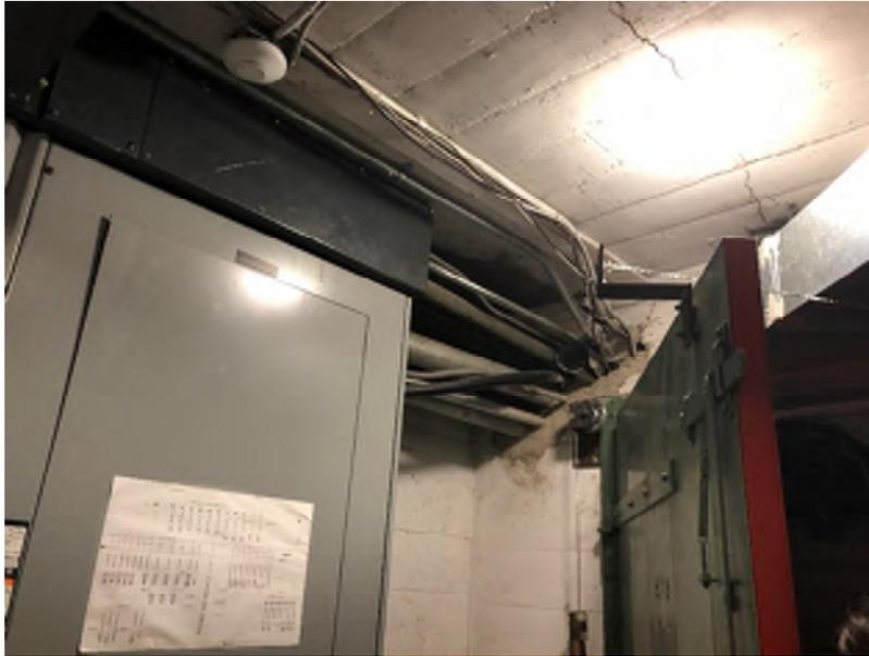
Typical Wiring without Fire Stopping
