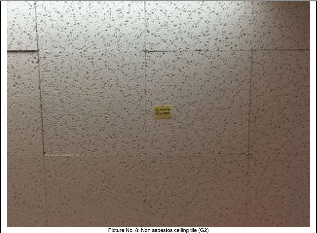
Picture No. 8: Non asbestos ceiling tile (G2)
