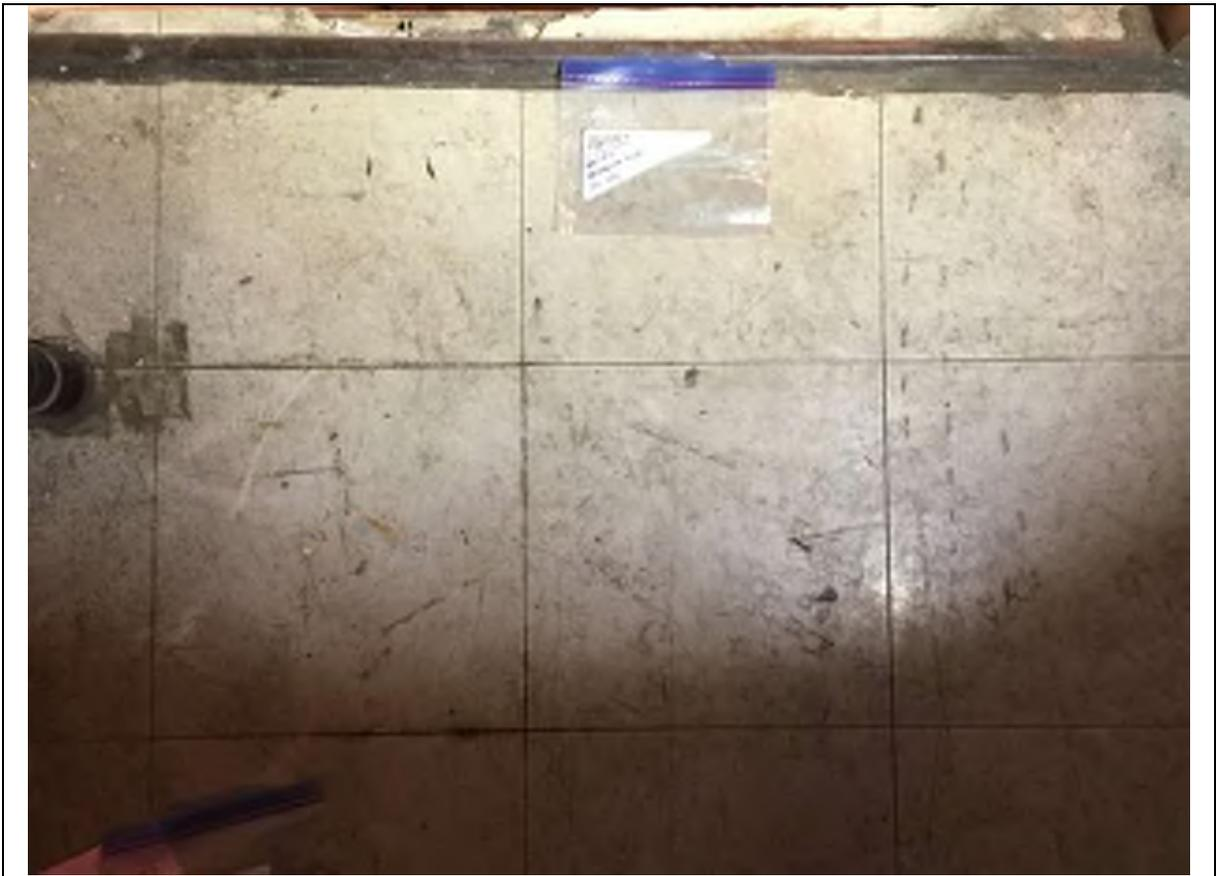
Picture No. 9: Non asbestos vinyl floor tiles (H2)
