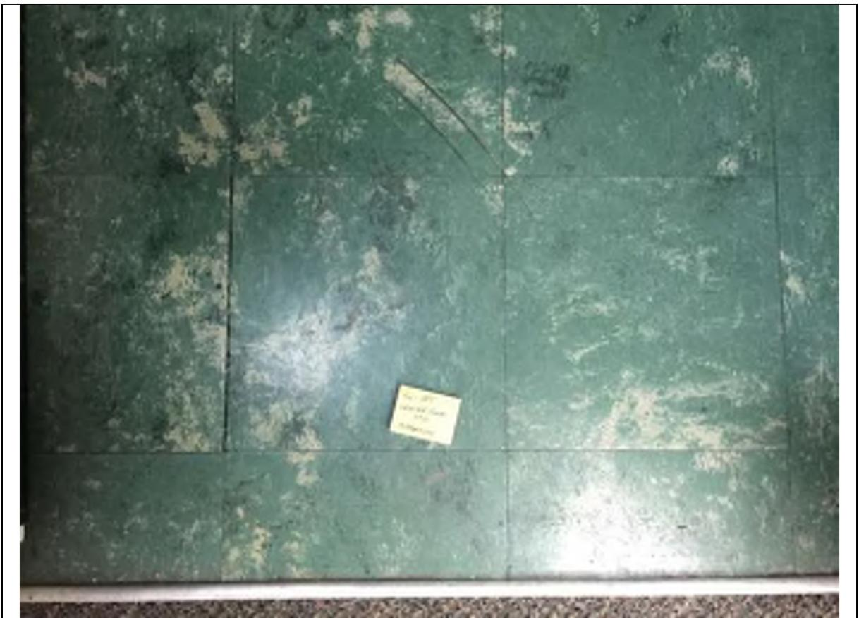
Picture No. 20: **Asbestos containing vinyl floor tiles (H4)**
