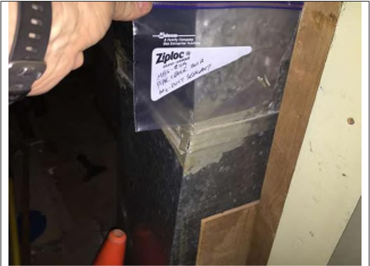
Picture No. 33: Non asbestos duct mastic (M2)
