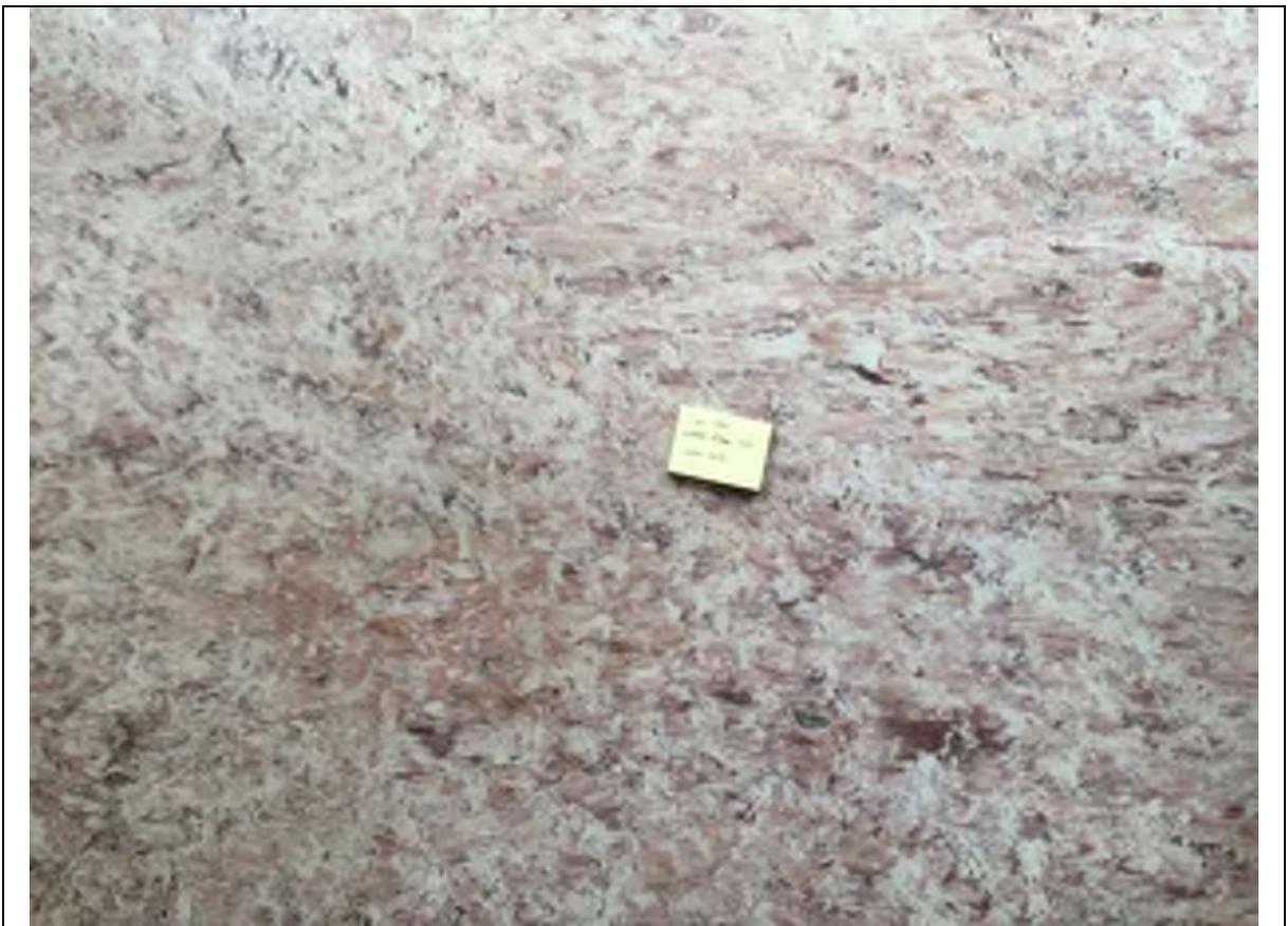
Picture No. 24: Non asbestos vinyl floor sheeting (I6)
