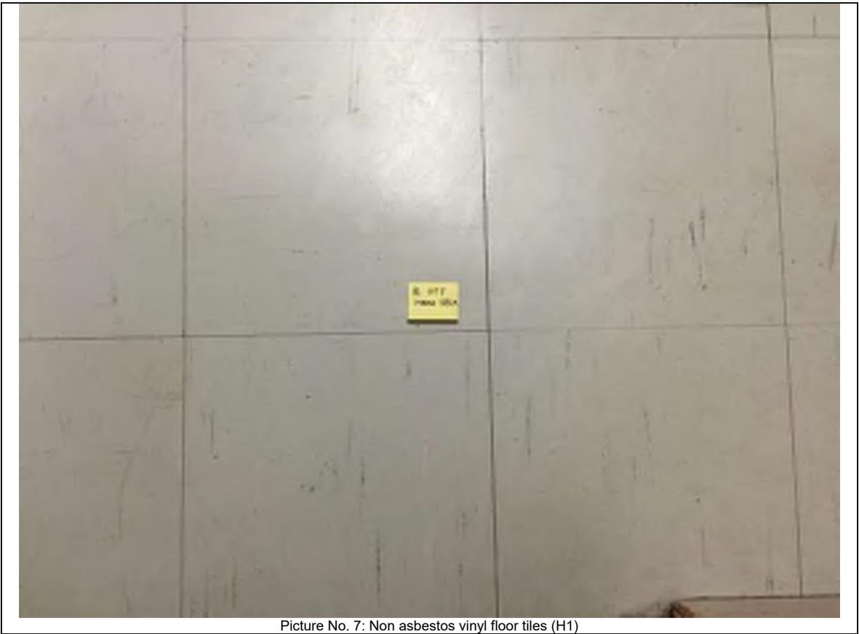
Picture No. 7: Non asbestos vinyl floor tiles (H1)
