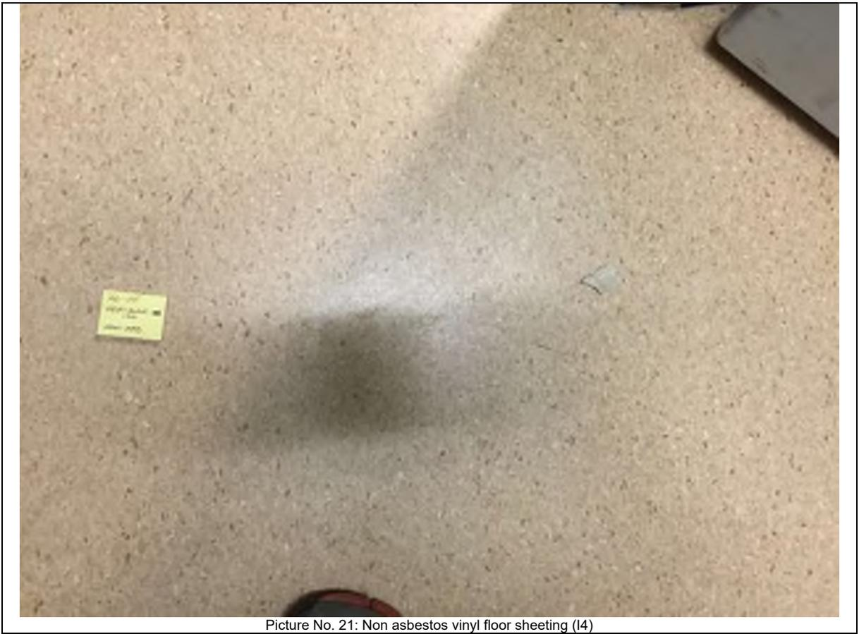
Picture No. 21: Non asbestos vinyl floor sheeting (I4)
