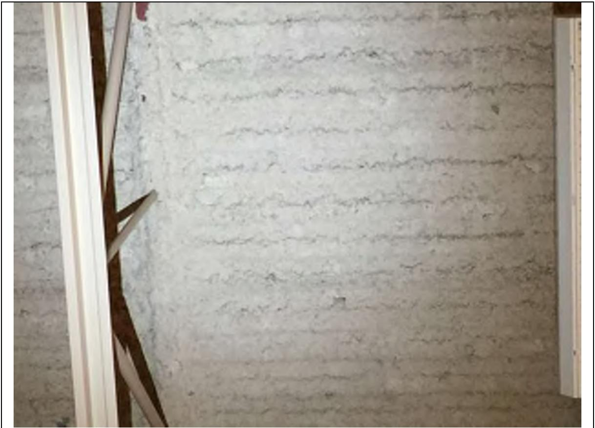
Picture No. 30: Suspect asbestos mastic on acoustic insulation (M5)
